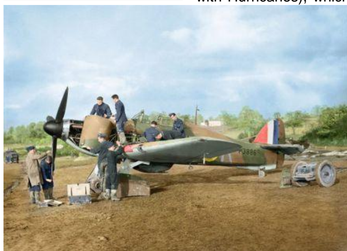
The feature image above shows "Hurricane Mk I UF-K of No 601 Squadron RAF while it is being serviced on the perimeter dispersal at RAF Exeter in mid-September 1940. This aircraft saw success with both Sgt Leonard N Guy and F/O Carl Raymond Davis.
